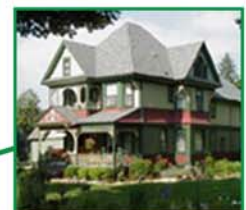
Habberstad House 706 Fillmore Ave S
